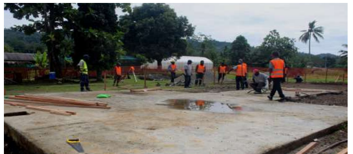
Phase 1 construction of the multipurpose shed.
