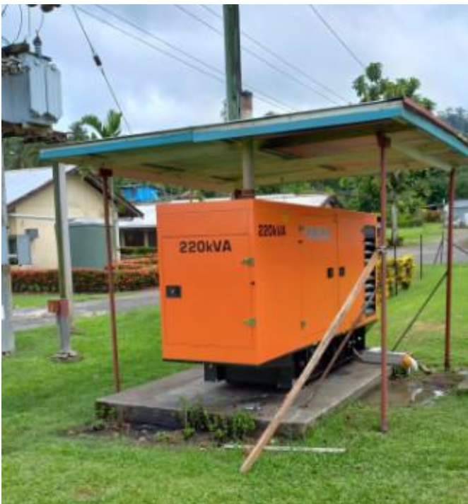
Figure 29: Bubia generator replacement
