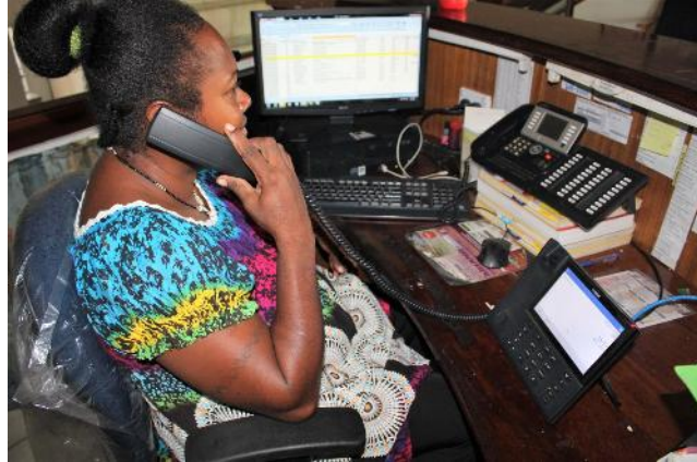
Figure 37: New VoIP PABX in operation at HQ Reception
