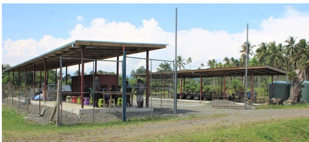
Figure 36: Rice field facility building at Bubia
