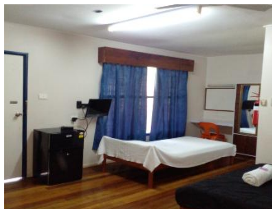
Figure 35: Guest house room renovation
