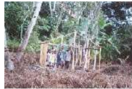
Constructing chicken house with local materials
