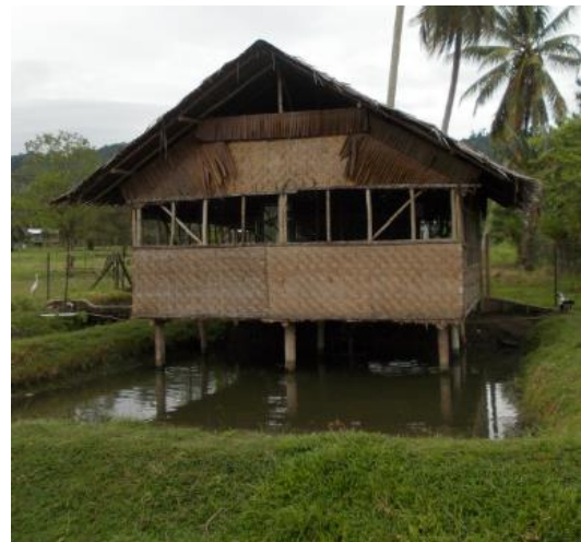
An integrated poultry unit built in front of the pond
