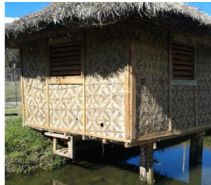
This house as part of its posts sitting on the bank of the pond while its other two posts are inside. There is also a widow for ventilation
