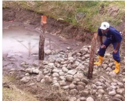
(2) Posts are placed into the pond with the bigger part of the house over hanging the pond
