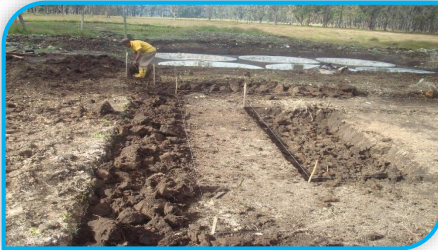
Figure 2. Fish pond constructed on a land that is relatively level
