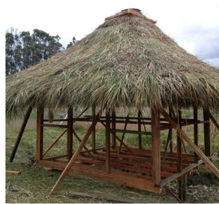
(4) The roofing goes first to keep the housing safe from the rain.
