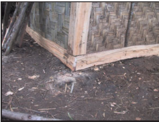
Bottom of wall buried and strengthened with timber to protect from dogs or other natural enemies
