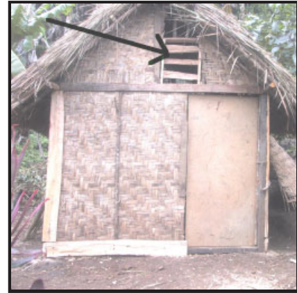
Bamboo wall with window
