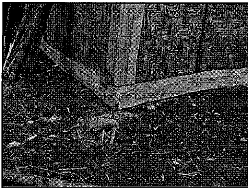
Bottom of wall buried and strengthened with timber to protect from dogs or other natural enemies
